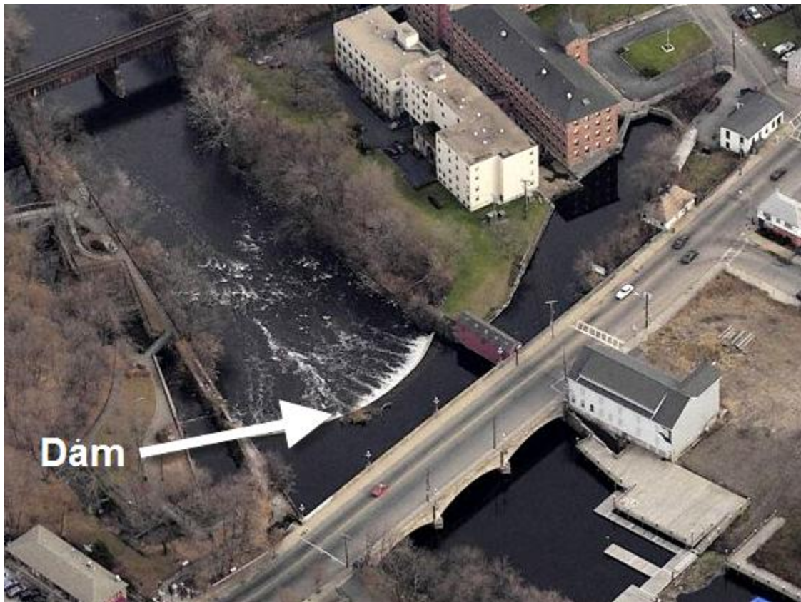
Figure 8 - Aerial Photograph of Valley Falls Dam (Flow from bottom right to top left)
